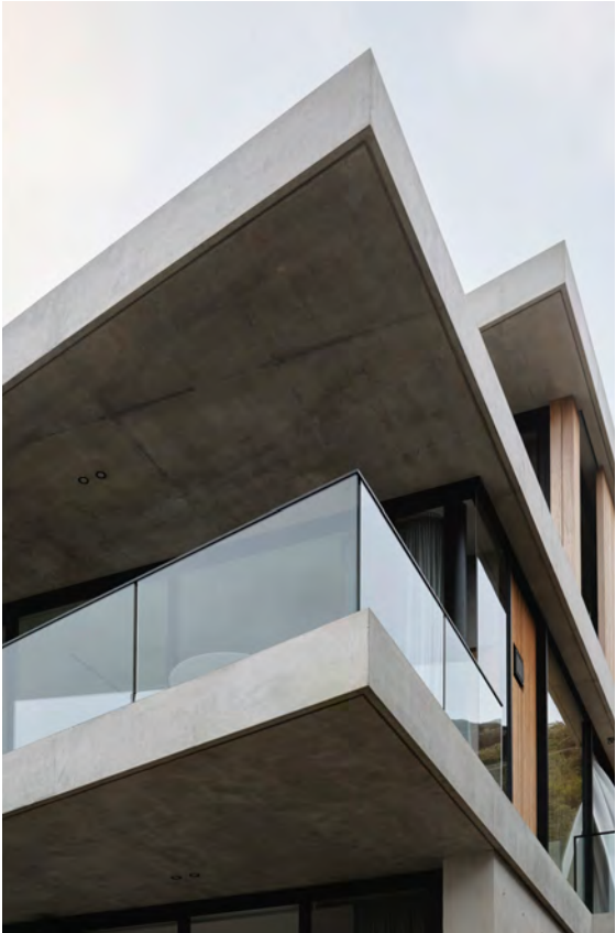
F02- OFF-FORM CONCRETE (SLABS)
